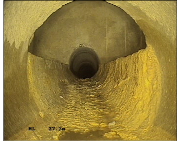
Photo: 8_2A, Media No.: 010208_1, 00:10:30 112FT, Downstream Manhole, Survey Ends
