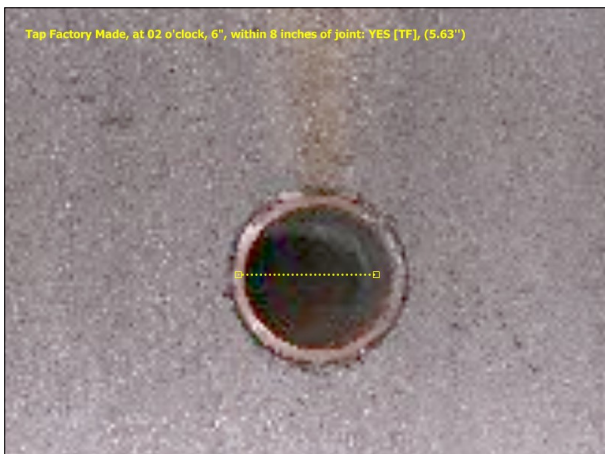
Photo: 7_4A, Media No.: 010208_1 105.97FT, Tap Factory Made, at 02 o'clock, 6", within 8 inches of joint: YES
