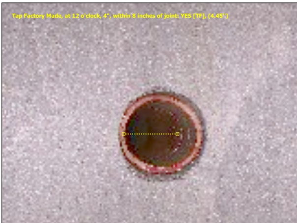
Photo: 7_2A, Media No.: 010208_1 29.73FT, Tap Factory Made, at 12 o'clock, 4", within 8 inches of joint: YES
