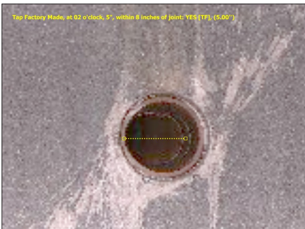
Photo: 7_10A, Media No.: 010208_1 244.04FT, Tap Factory Made, at 02 o'clock, 5", within 8 inches of joint: YES
