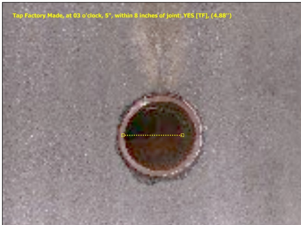
Photo: 7_3A, Media No.: 010208_1 90.59FT, Tap Factory Made, at 03 o'clock, 5", within 8 inches of joint: YES
